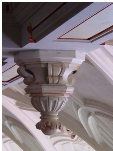
Photo 3 Rehabilitation of Paintings in Main Waiting Room
