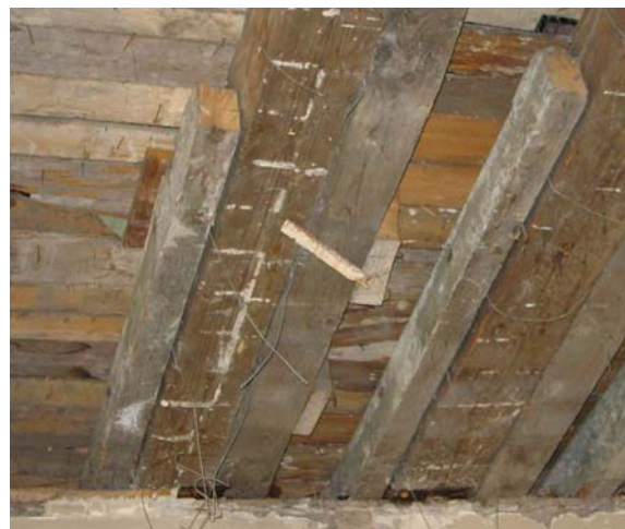
Photo 4 Replacement of wood floors in superstructure
