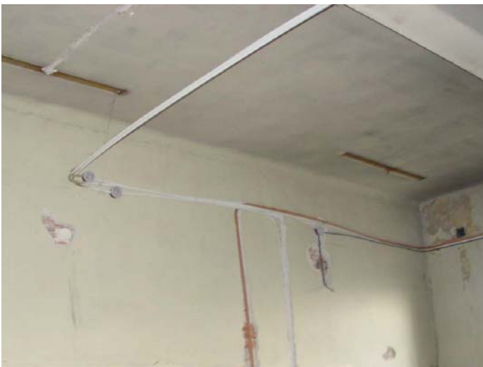
Photo 6 New Compartment and Installations
