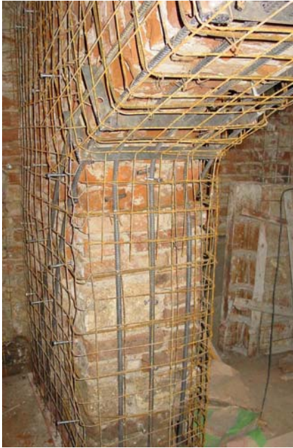
Photo 1 Alba Iulia Railway Station – Infrastructure’s Rehabilitation
