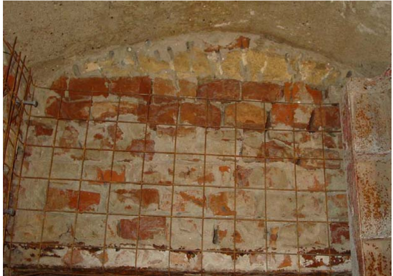
Photo 2 Alba Iulia Railway Station - Infrastructure’s Rehabilitation
