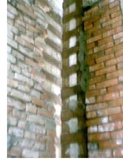
Photo 11 RC Pillars at Walls' Intersections
