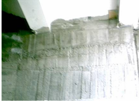
Photo 10 Supplementary structural wall
