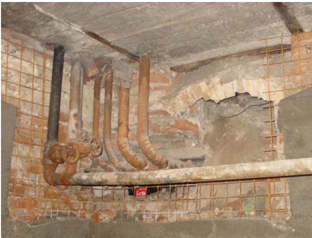
Photo 3 Alba Iulia Railway Station- Infrastructure’s Rehabilitation of Installations
