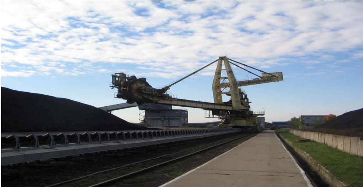
Fig. 4 The rail roads and machine
