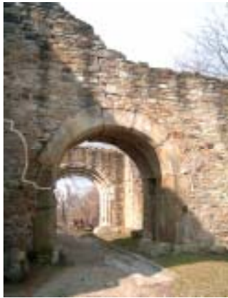
Main split in the reconstructed vault
