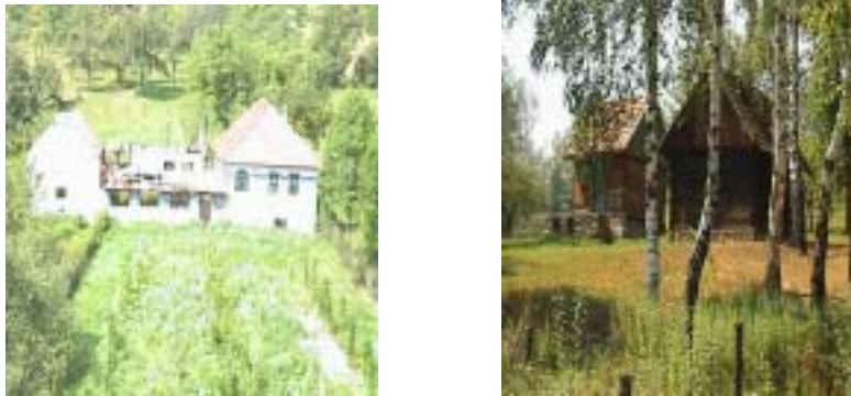
Fig 1 Constructions affected by the mining exploitation from Maleia zone
