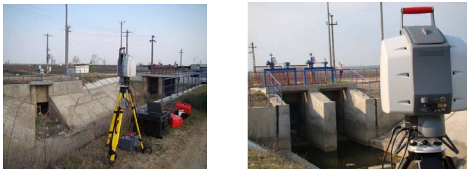
Fig. 3. The laser scan ready for action
