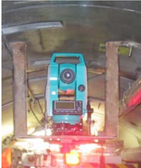
Fig.6.Positioning the total station in the work axis
