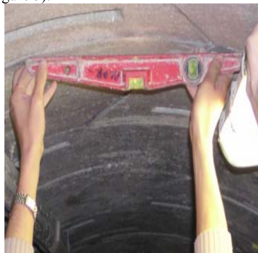
Fig.5 Positioning the laser support
