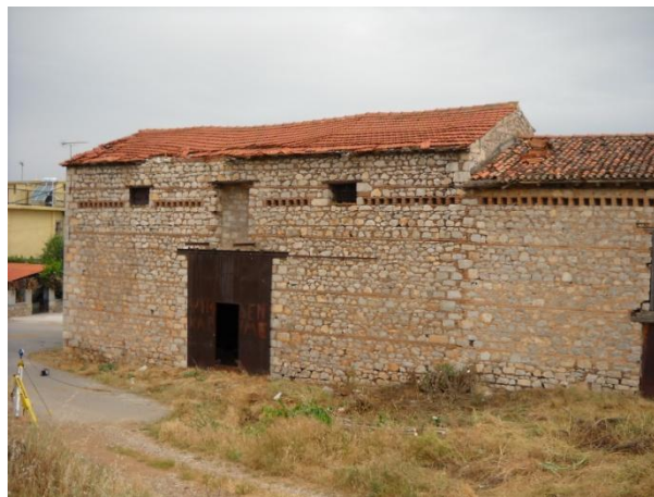
Figure 2: Photograph of the industrial building in Thiva area
