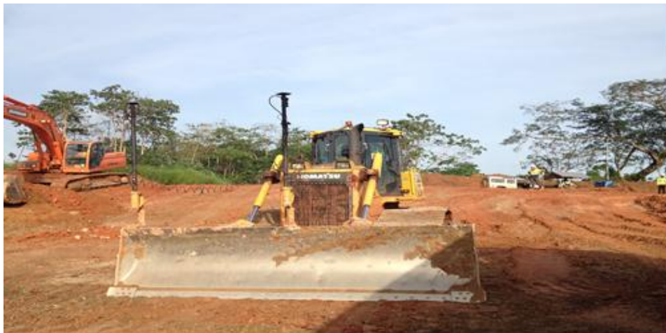
Fig. 11. Machines equipped with GPS technique (automatic control)
