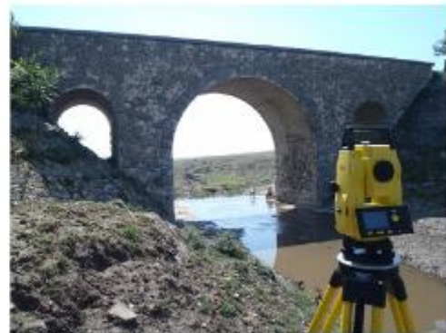
Figure 2 – Railway Bridge Targusor
