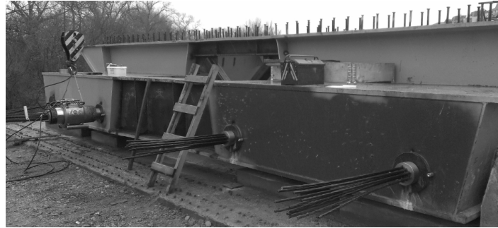
Fig. 7. The prestressing process
