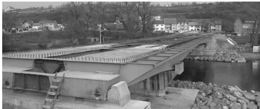
Fig. 5. Encasements filled with reinforced concrete
