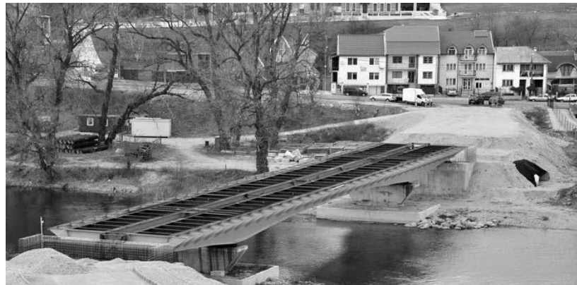
Fig. 4. Initial state of the metallic superstructure
