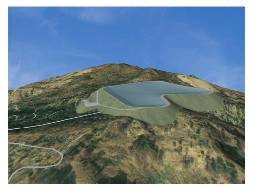
Figure 19. Area 3 - proposed upper reservoir 2.8 Mm<sup>3</sup>
