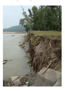
Figure 6 Degradation of left shore protection works of Moldova River after floods in 2010
