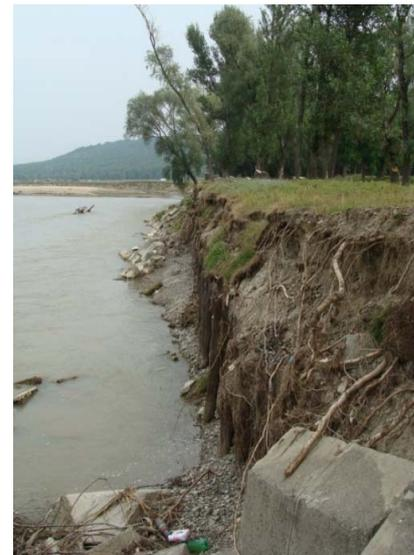
Figure 6 Degradation of left shore protection works of Moldova River after floods in 2010
