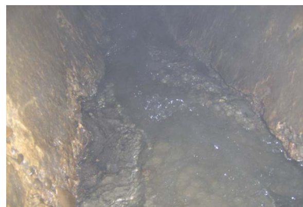
Fig. 1. Degradation of the flow section through silted accessible sewer drains; a- cemented silting; b - silting during concentration and cementation.
