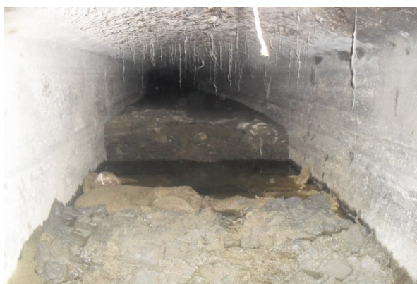
Fig. 1. Degradation of the flow section through silted accessible sewer drains; a- cemented silting; b - silting during concentration and cementation.
