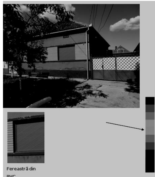
Fig. 3. House – type 2 Well maintained building, plastered, old rooftop
