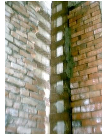
c. Reinforced concrete pillars at the intersection of load-bearing walls
