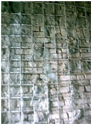
a. Underpinning foundations
