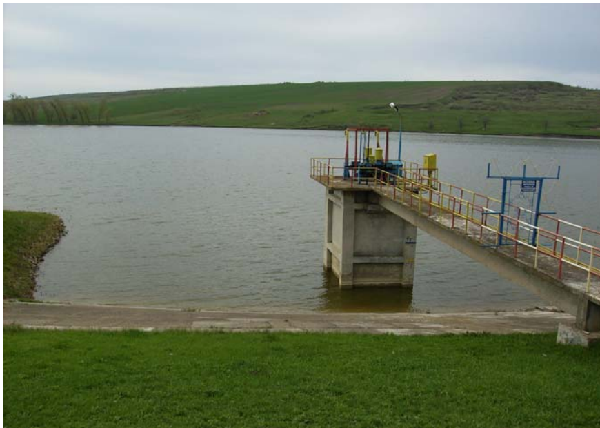
Fig.1. The barrier lake Cucuteni – Water Basinal Administration Prut-Barlad
