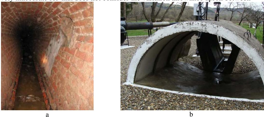
Fig. 4. Profile sewer visitable collectors modified; a - type ovoid; b - semi-elliptical bell.
