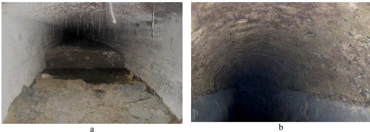
Fig. 1. Degradation one flow path to the sewage collectors visit; a - clogging invert and cementing material deposits; b - the degradation of concrete soffit plate coverage to a collector type ovoid.
