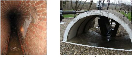
Fig. 4. Profile sewer visitable collectors modified; a - type ovoid; b - semi-elliptical bell.
