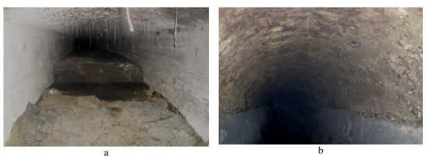
Fig. 1. Degradation one flow path to the sewage collectors visit; a - clogging invert and cementing material deposits; b - the degradation of concrete soffit plate coverage to a collector type ovoid.
