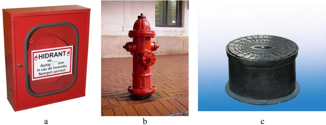
Fig. 2. Types of hydrants used in localities: a - hydrant box inside the building; b - surface hydrant; c - underground hydrant
