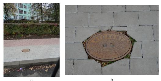
Fig. 3. Street underground hydrant: a - general view; b - detail, the hydrant box.
