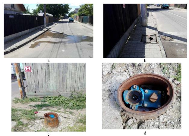
Fig. 7. General view and details of the status of street hydrants: a - general view of Ceahlău street, Iași city; b - general view Aurel Vlaicu street, Iași city; c - the location of the underground hydrant; d - details of the hydraulic installation in the hydrant box.
