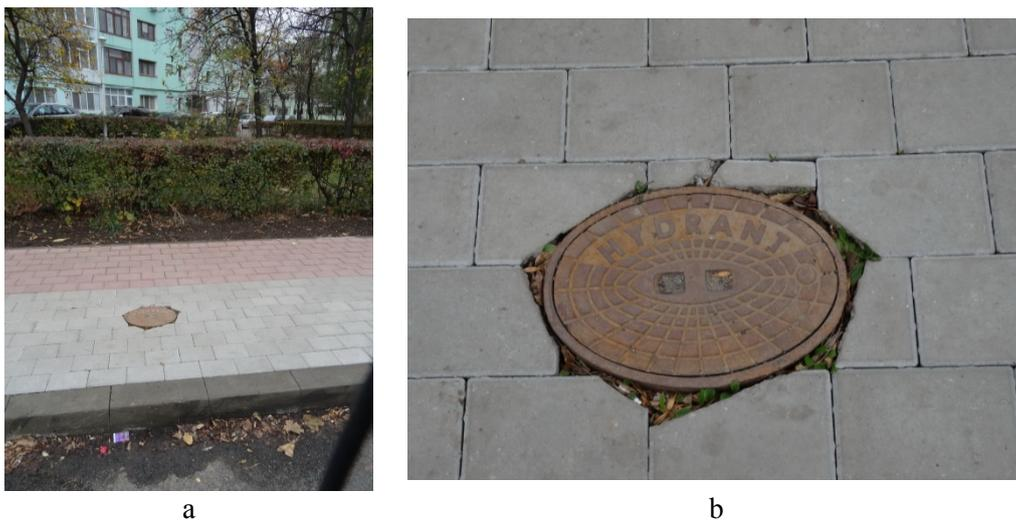
Fig. 3. Street underground hydrant: a - general view; b - detail, the hydrant box.
