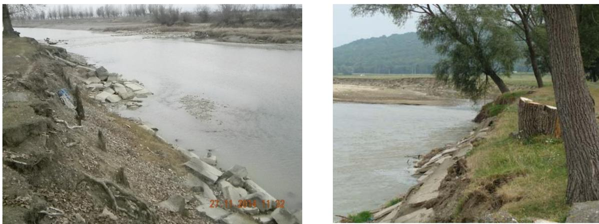
Fig. 7. Details of the erosive water action on the left bank of the river Moldova upstream of the undercrossing of the adduction pipelines: a - defence of total degraded river (2012); b - left eroded with the collapse of shore defence (2012) (Luca M., 2012a).
