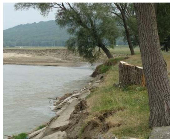
Fig. 7. Details of the erosive water action on the left bank of the river Moldova upstream of the undercrossing of the adduction pipelines: a - defence of total degraded river (2012); b - left eroded with the collapse of shore defence (2012) (Luca M., 2012a).
