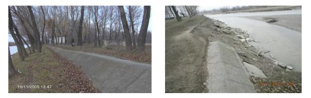
Figure 5. General view of the evolution of Moldova's river bank to the effects of floods: stable in 2005; b - eroded in 2012 (Luca M., 2016).
