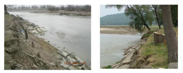
Fig. 7. Details of the erosive water action on the left bank of the river Moldova upstream of the undercrossing of the adduction pipelines: a - defence of total degraded river (2012); b - left eroded with the collapse of shore defence (2012) (Luca M., 2012a).
