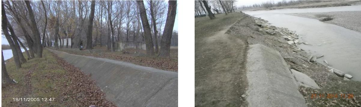
Figure 5. General view of the evolution of Moldova's river bank to the effects of floods: stable in 2005; b - eroded in 2012 (Luca M., 2016).
