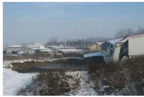
Fig. 5 Initial cone edge, Ocna Mures
