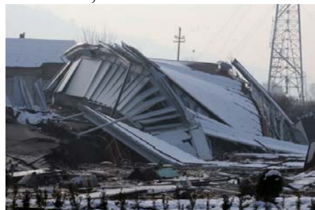
Fig. 7 “Plus” Supermarket during the collapse, Ocna Mures
