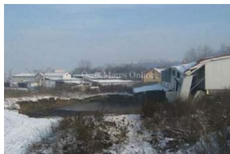
Fig. 5 Initial cone edge, Ocna Mures
