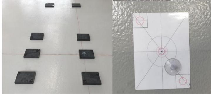
Fig. 4 Using the Chalk Line and the Template
