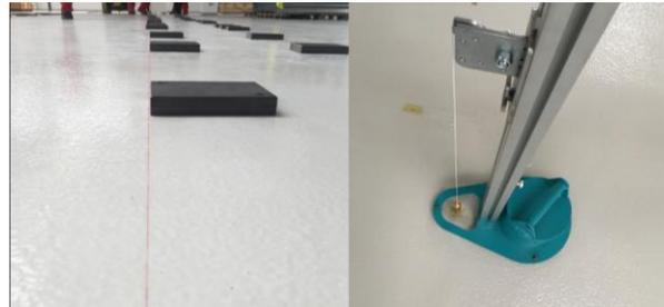
Fig. 5 Using the lead wire and chalk line
