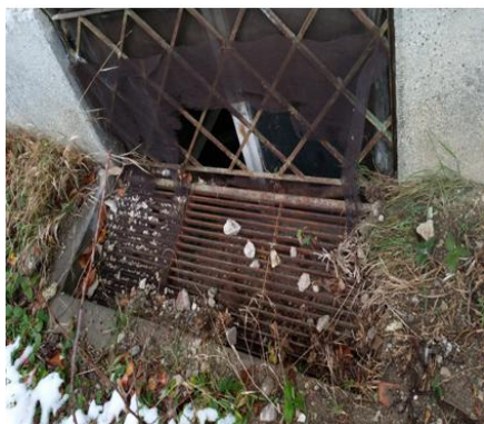
Fig.5 Position the windows in the basement
