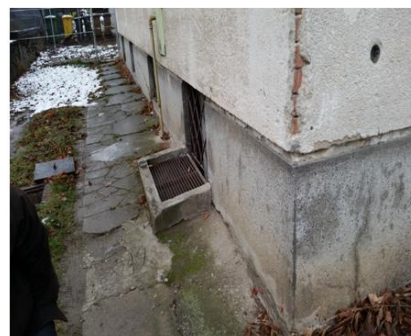
Fig.4 The front side pavement
