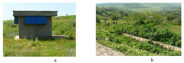
Fig. 4. Location type of the adduction pipes interventions: a - permanent location, valve chamber on the adduction AdIIa + AdIIb; b - random location, failure on AdI adduction (Luca, 2015).
