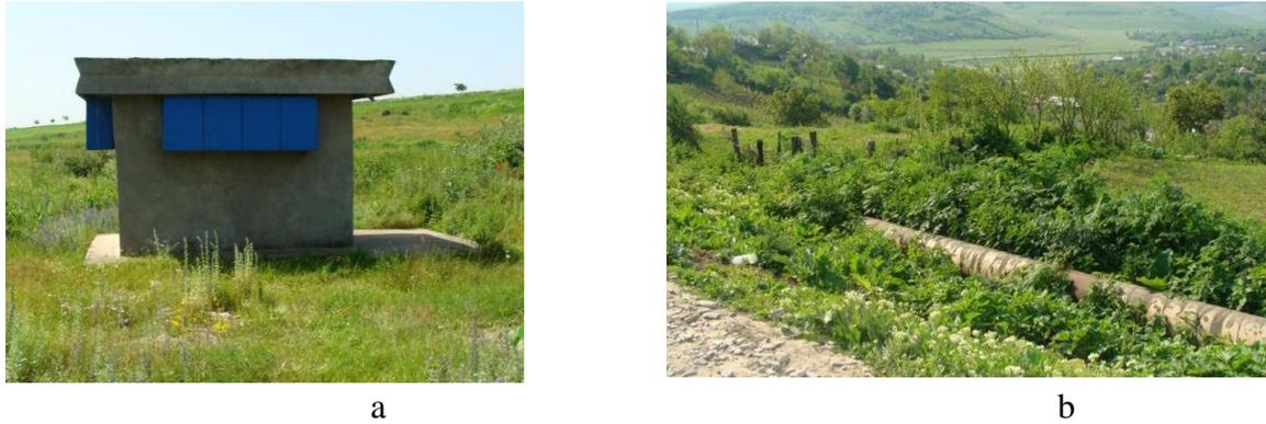
Fig. 4. Location type of the adduction pipes interventions: a - permanent location, valve chamber on the adduction AdIIa + AdIIb; b - random location, failure on AdI adduction (Luca, 2015).
