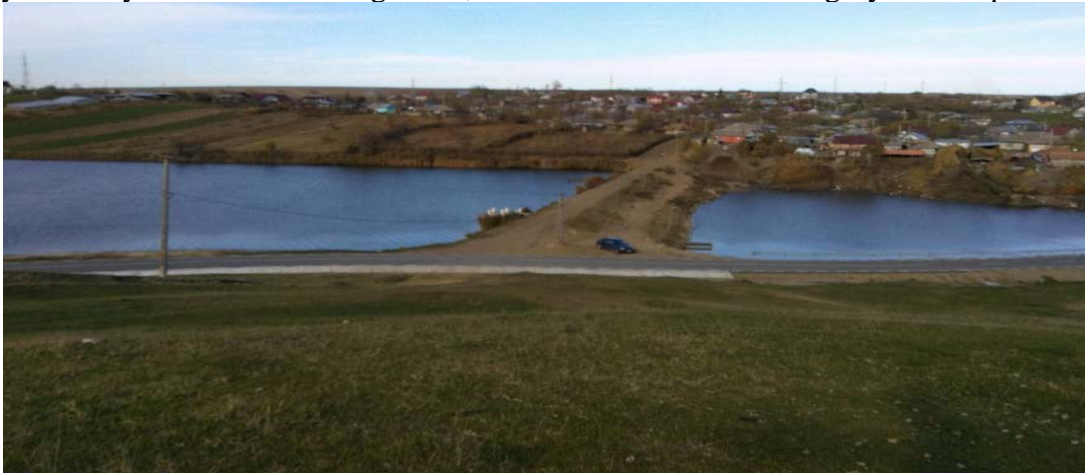
Figure 3 – General view of the Podisu dam (source: author)
