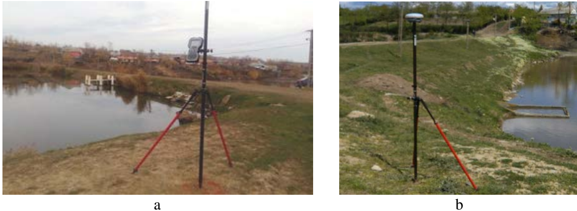
Figure 11 – The condition of the slopes at Podisu dam in 2021: a – upstream slope; b – downstream slope (source: author).
