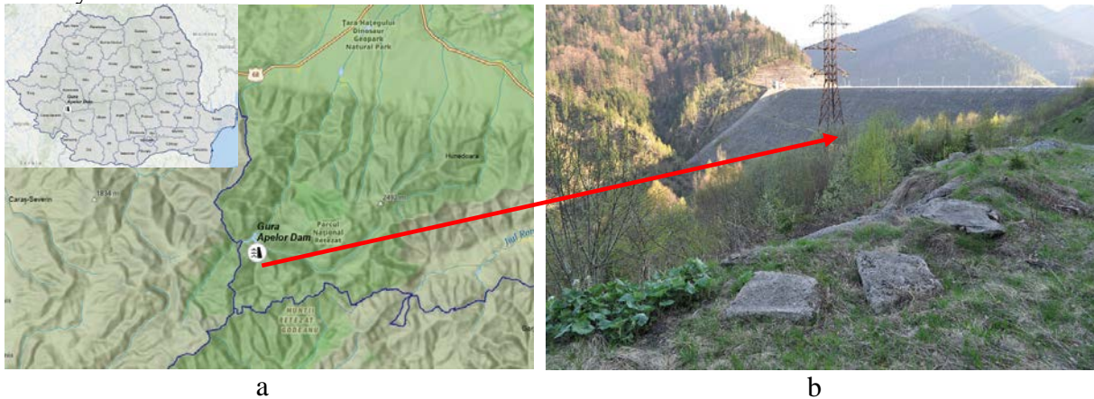
Figure 1– Gura Apelor Dam: a - study area location on the map of Romania and the map of Retezat National Park; b - downstream view of the dam.
