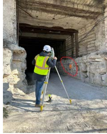
Fig. 3. Measurements with Leica Viva TS15 total station
