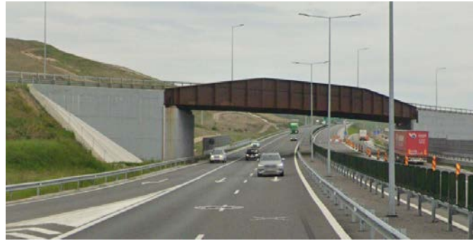
Figure 2: National road DN 1 over the A10 highway
