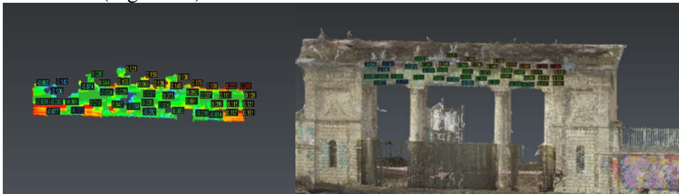
Figure 13. Deviations of the upper wall of the stadium entrance gate
